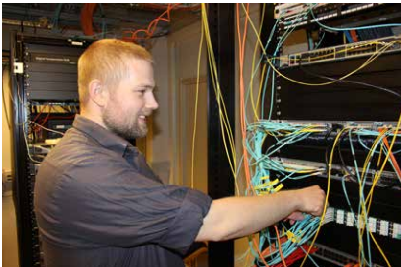
Left: Kim Eirik Kvasheim inspecting cables
